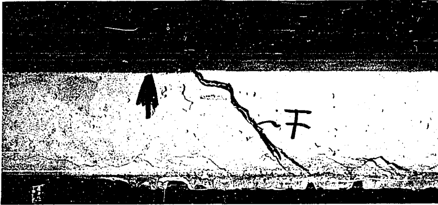
Fig. 13. Typical shear-bond failure crack of beam constructed with steel deck I. Arrow indicates point of load application
